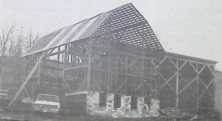
In photo above and to the right, one of the Shell brothers climbs among the beams of the reassembled barn. The photo above and to the left and the one below show the barn as it has been incorporated with existing buildings. Space for a workshop was made under one end of the barn, and fiberglass panels were added to the roof for lighting.
