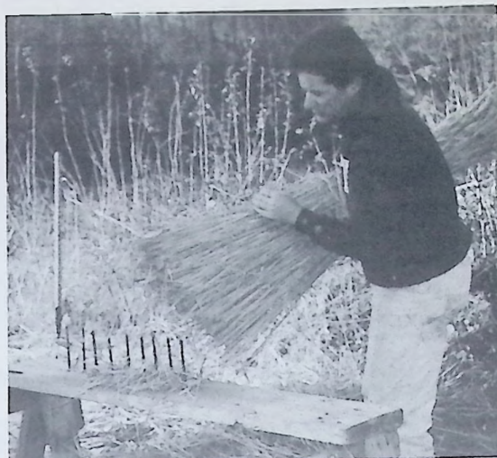
Mark Powell of County Cork, Ireland, combs and straightens rye straw for placement on the thatched roof of a farmhouse at the Museum of American Frontier Culture.
